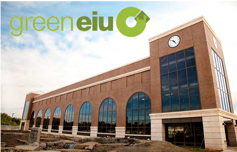
Eastern's Renewable Energy Center
